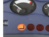
Lifting interlock lamp on the control panel
